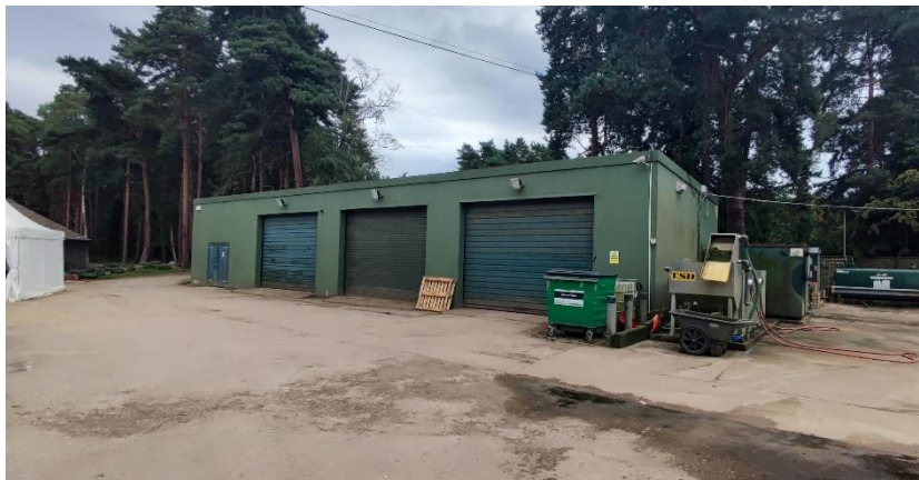
Existing building D (to be demolished) and service vehicles stored outside
